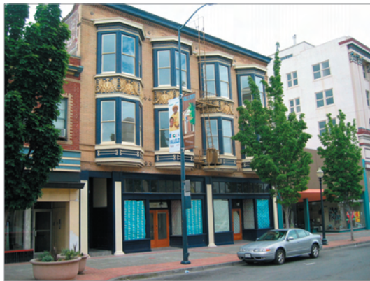
Figure 3.C.78: Bays, recesses and overhangs break up the building's facade to create a dynamic frontage.
