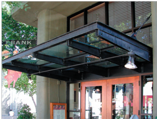
Figure 3.A.41: Glass and metal canopy complements the contemporary architecture of this building and provides protection from rain at the building entrance.
