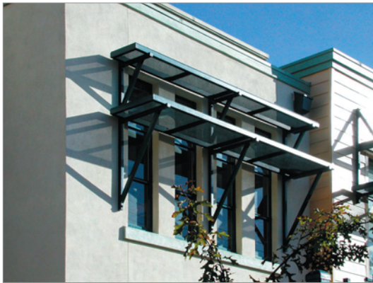
Figure 3.A.38: Architectural canopies shade a window while creating attractive articulation on a building façade.
