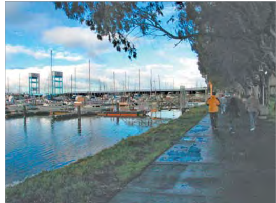
Figure 3.D.6: View Across Marina to Causeway Bridge
