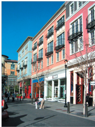
Figure 3.C.81: Facades with simple massing are balanced by a series of Juliet balconies that create a human-scaled connection between upper floors and the street.
