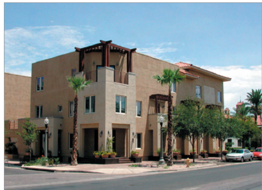
Figure 3.A.24: (Example of Poor Design) Roofs that are devoid of interest create abstract buildings that are less engaging to pedestrians.
