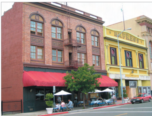
Figure 3.C.59: A Well-Defined Building Wall.
