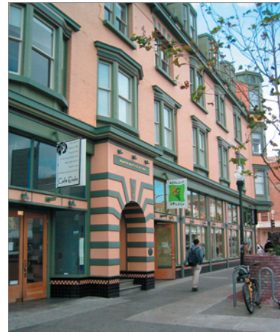
Figure 3.A.29: A well articulated primary residential entry is made distinct from storefront entries with color, change in materials and articulation.
