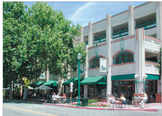
Figure 3.C.62: Parking garages can be designed to support a high-quality pedestrian environment
