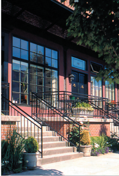
Figure 3.A.31: Attractive Residential Stairs
