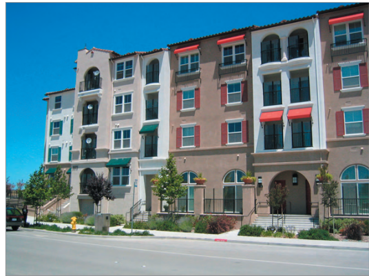
Figure 3.B.44: Poor Example of Rooflines - Not Enough Relief or Variation
