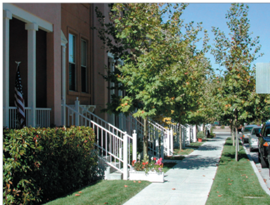
Figure 3.A.5: Residential uses should front sidewalks with primary entrances that incorporate porches, stoops, stairs, and the more active interior spaces.
