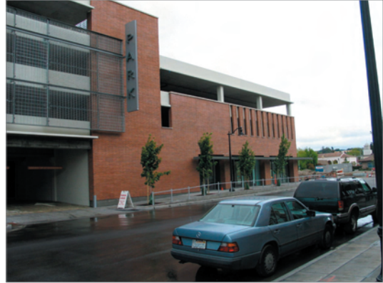
Figure 3.C.67: (Example of Poor Design) Excessive blank walls along a parking garage creates an uninviting and inactive street frontage and should be avoided.
